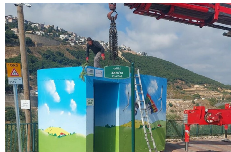
A painted bomb shelter being installed in the local Druze community, Hurfeish (photo: Operation Lifeshield)
